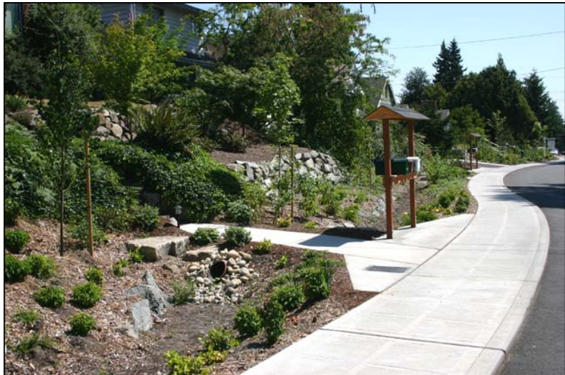
A drainage swale runs along the length of the sidewalk to capture and slow storm runoff from paved surfaces.
