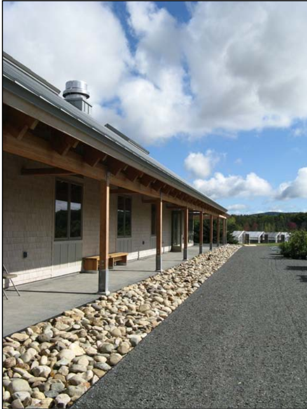
An infiltration trench captures sheet flow off the roof of a facility at Nasami Farm in Whately.
