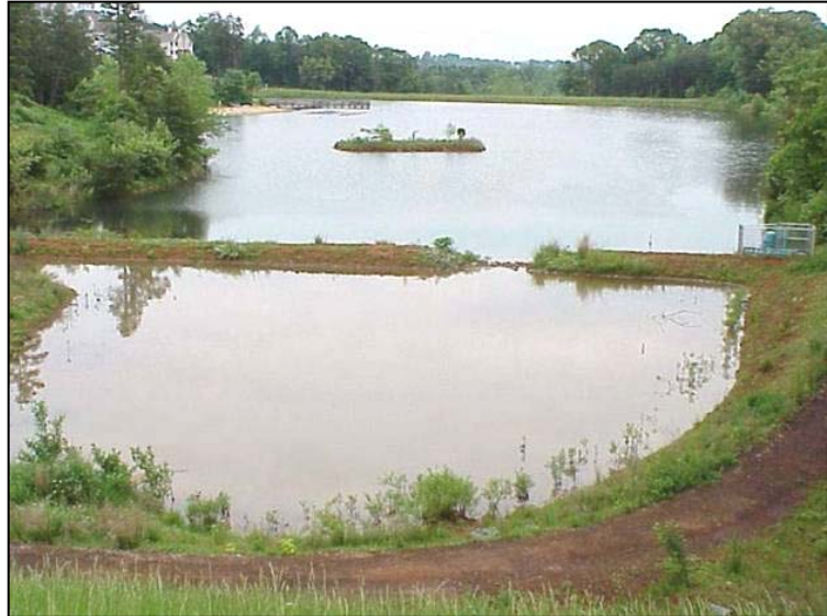
A sediment forebay slows flow so sediment can settle out before water moves to the main pool. Image courtesy Virginia Tech.
