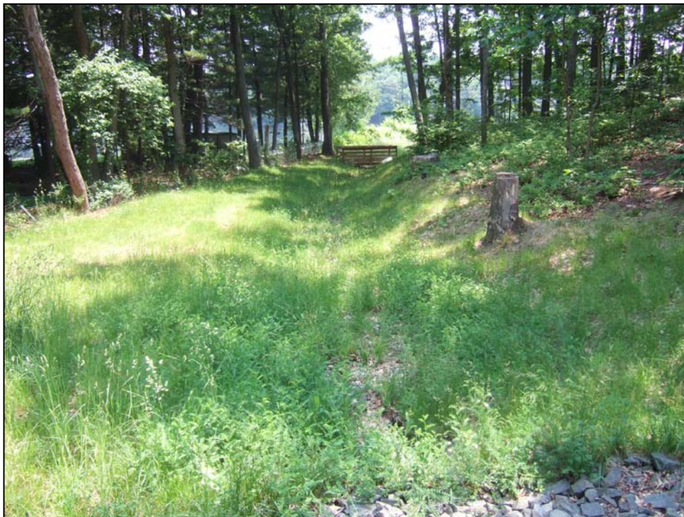
Vegetated swale drains to outfall at lake. Pedestrian footbridge provides access over swale to public picnic area.
